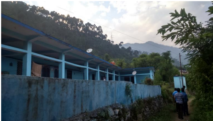
HOUSES HAVING DISH ANTENNAS
