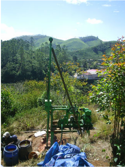
Fig. 16 Drilling machine at L 3
